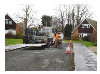
The asphalt slurry is mixed from liquid bitumen, fine aggregate, cement and chemicals.
