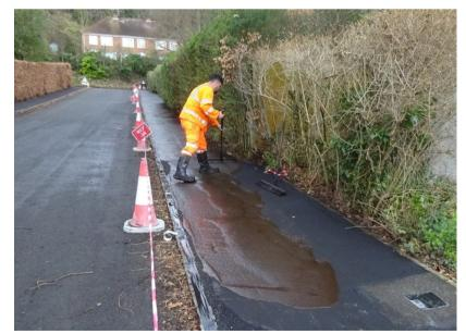
The slurry is spread by hand, in two consecutive layers.
