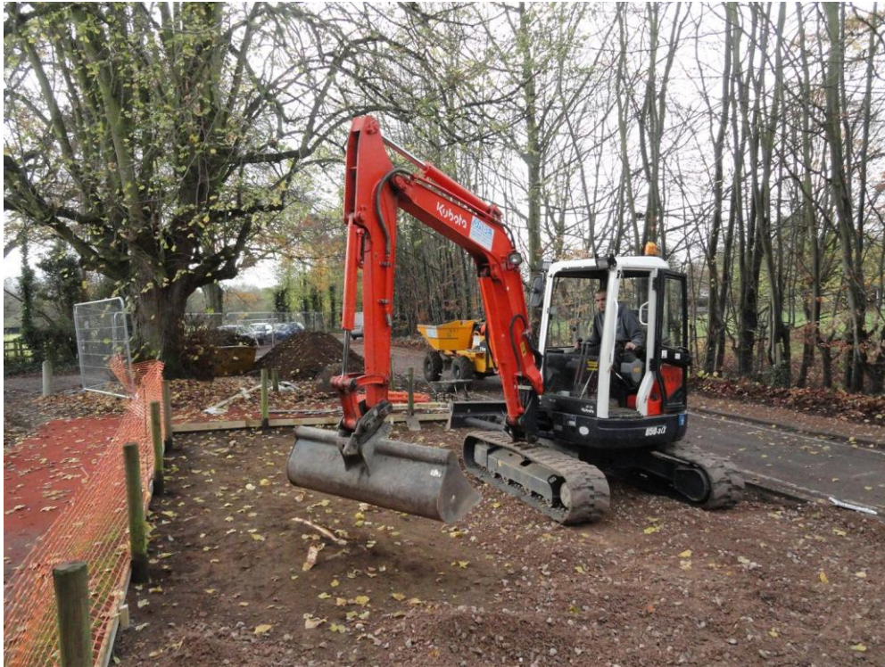
School car park under construction
