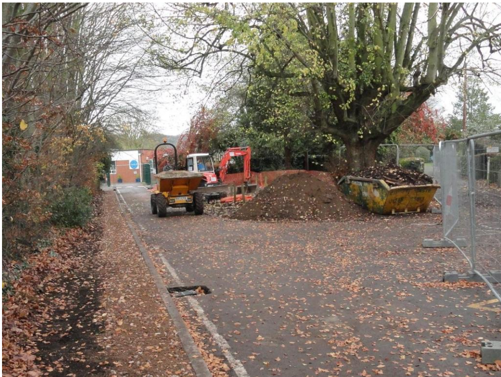
New gravel drain under footway (left) and an extra soakaway
