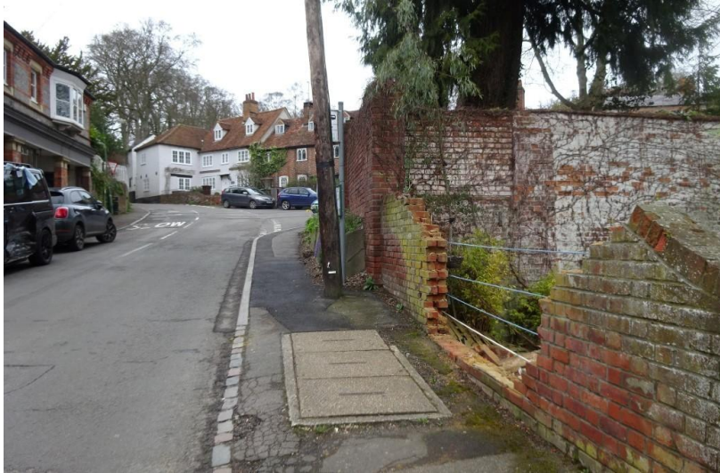
Seen here is the latest case of damage to a High Street brick wall caused by a vehicle out of control
